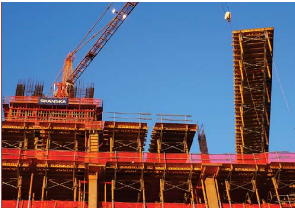
Flying table forms for the accelerated construction of the tower slabs.
