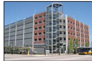
Renton Parking Garage Renton, Washington
